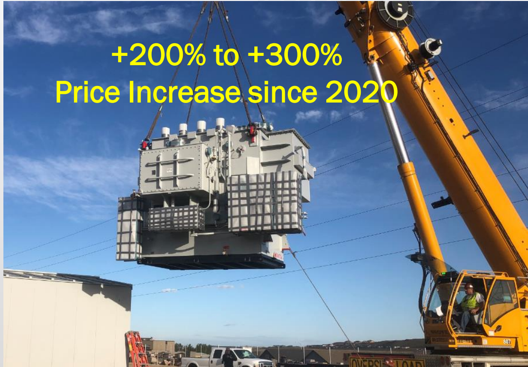
25-megawatt Substation Transformer
