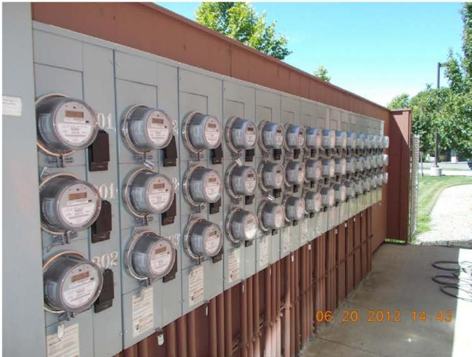
**Figure 8.** Large smart meter bank consisting of 45 meters at a retirement apartment complex. The meters face an adjacent apartment.
